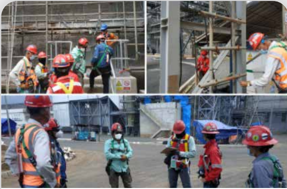
Inspeksi Onshore di Absorber 2 Onshore Inspection in Absorber 2
