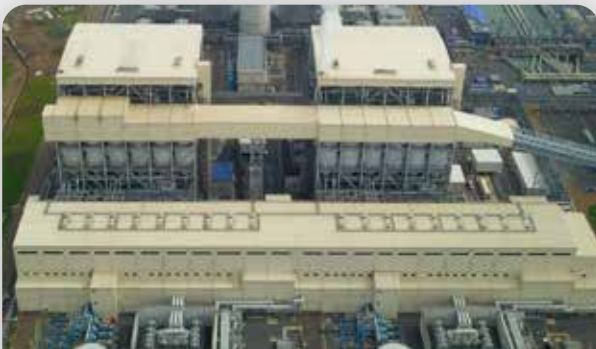
Turbin Unit #1 & Unit #2 Turbine Unit #1 & #2
