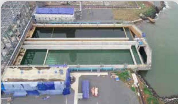
Kolam Aerasi Aeration Basin
