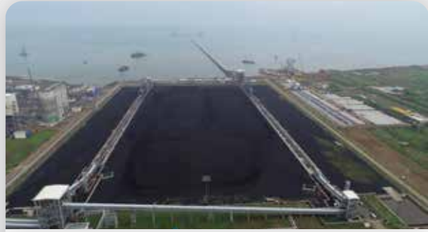
Area Penimbunan Batu Bara Coal Yard Area
