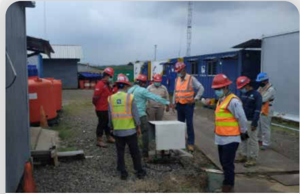
Inspeksi Onshore di Workshop dan Site Office Onshore inspection at Workshop & Site Office
