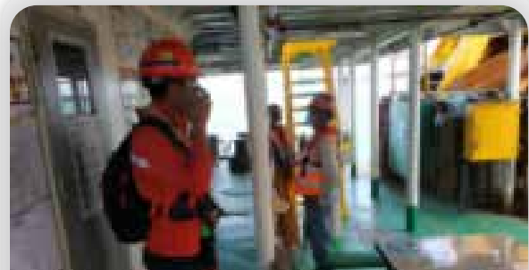
Inspeksi Offshore Offshore inspection
