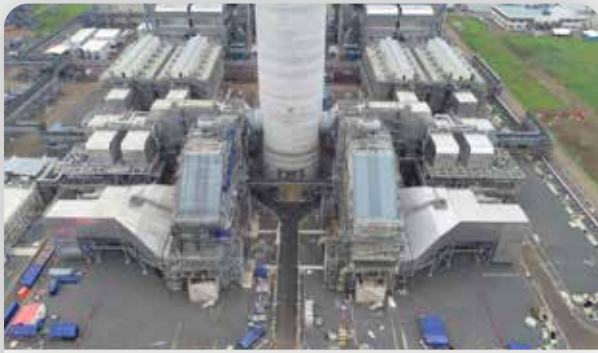
Peralatan Absorpsi Unit #1 dan Unit #2 Absorber Unit #1 & Unit#2
