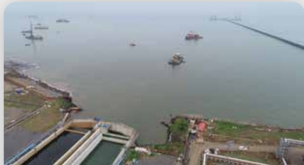
Pipa Pembuangan Air Bahang Cooling Water Pipe Outfall Line
