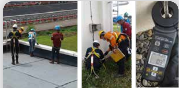
Inspeksi Penyalur Petir di Gedung Area IPAL Inspection of Lightning Protection at WWTP Building
